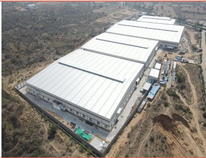
Exhibit 11: KRN HVAC new Facility -75K Sq mt.
