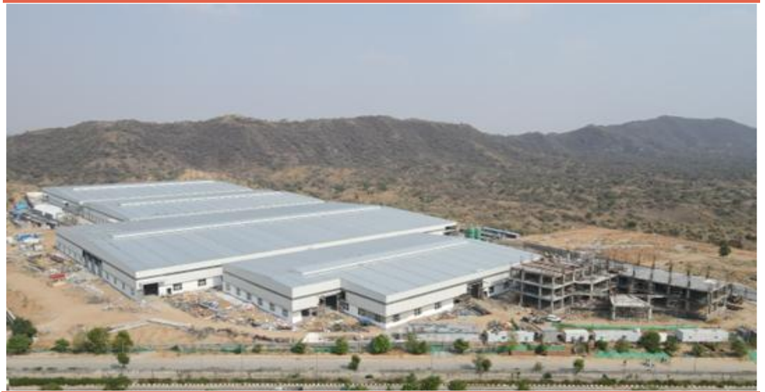
Exhibit 13: Full commissioning of new facility by Sept 2025; covered area – 0.6mn sq. ft.
